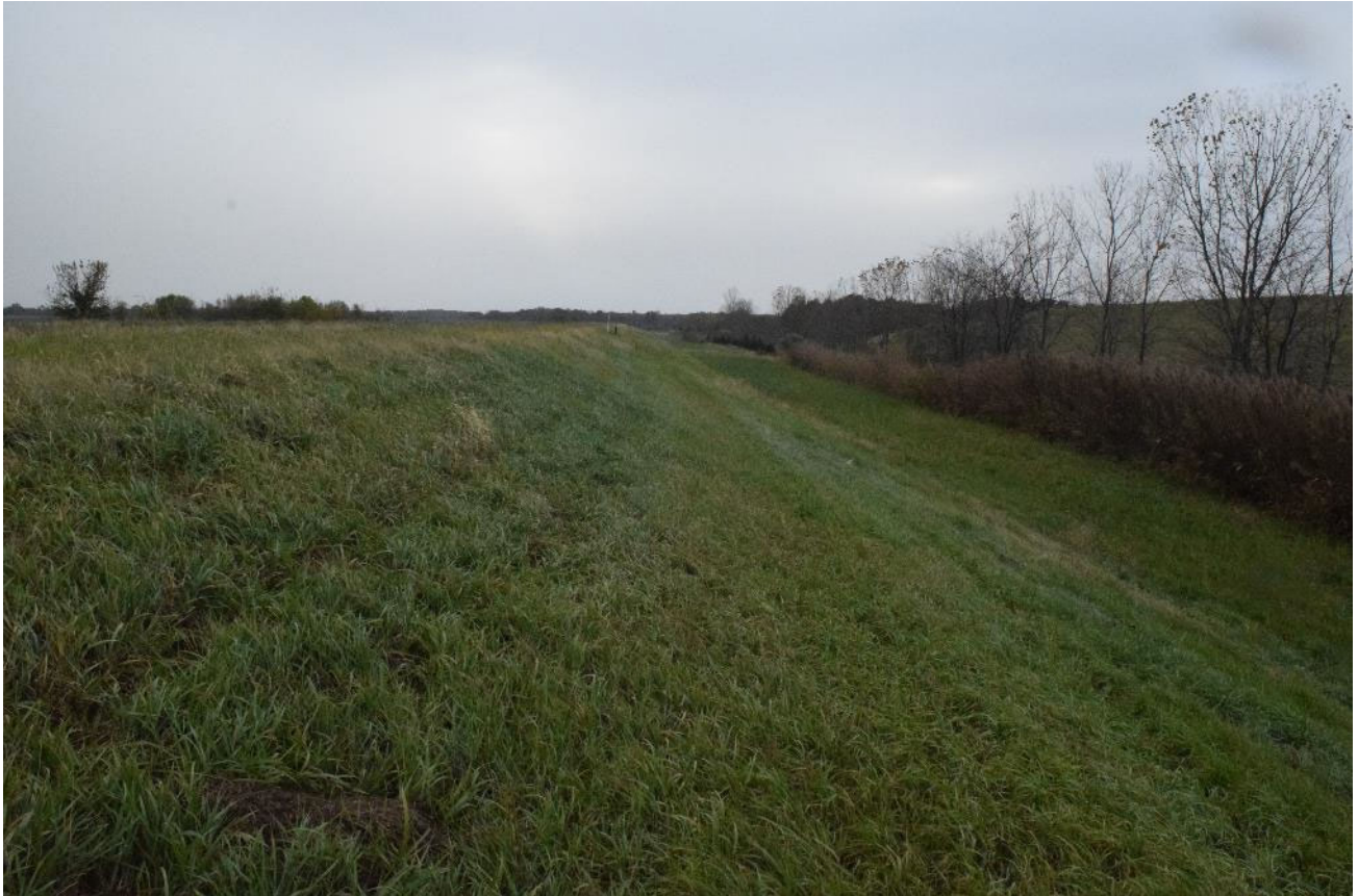
West downstream slope
