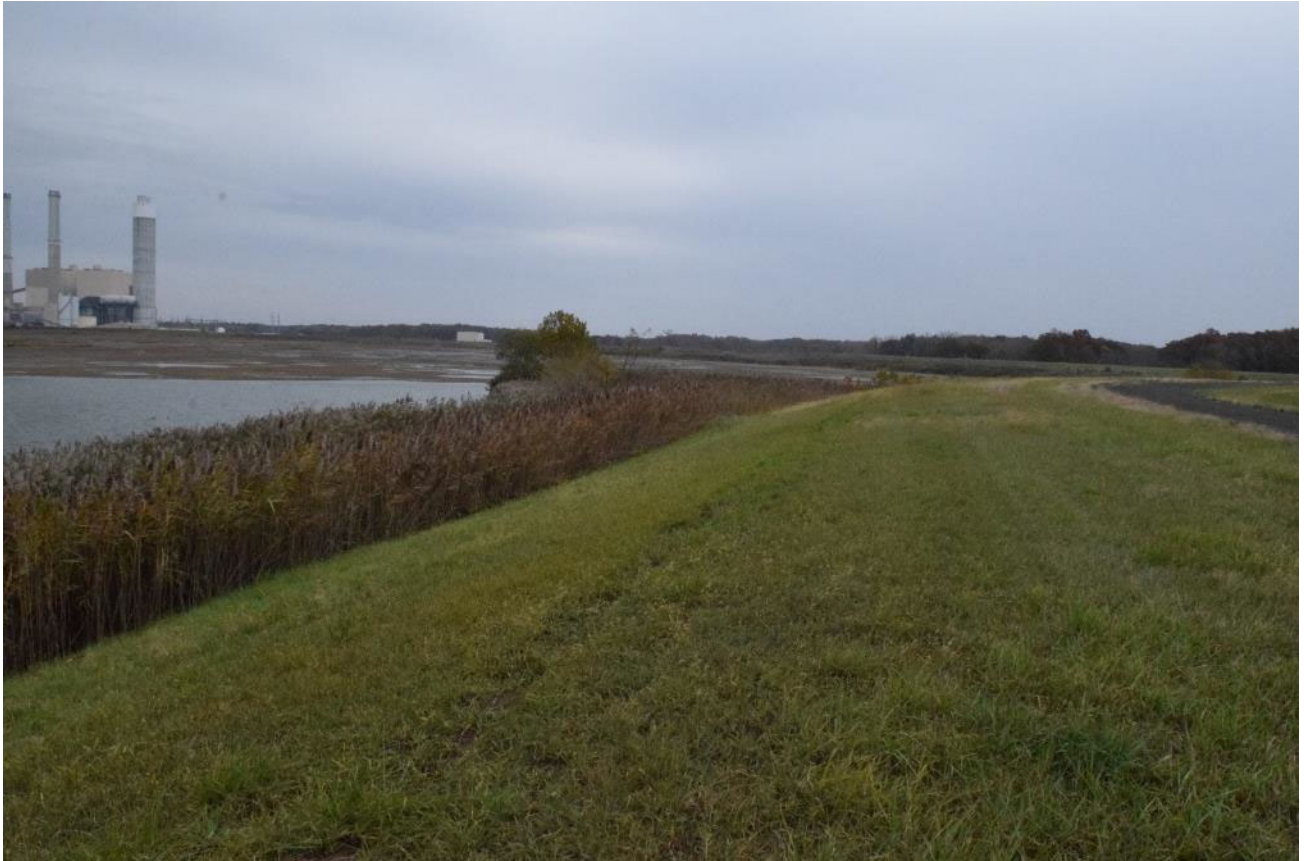
East crest and upstream slope
