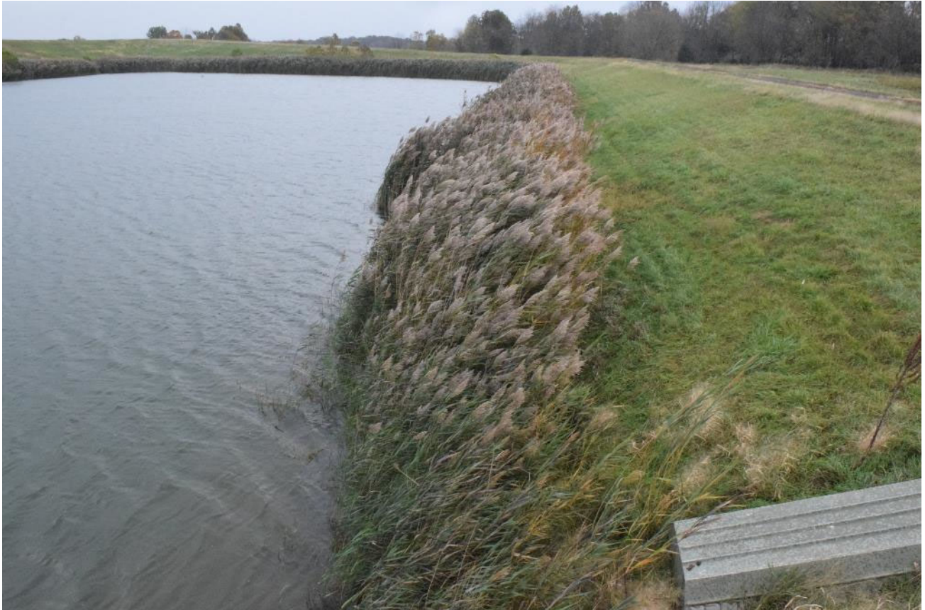
Interior of secondary pond
