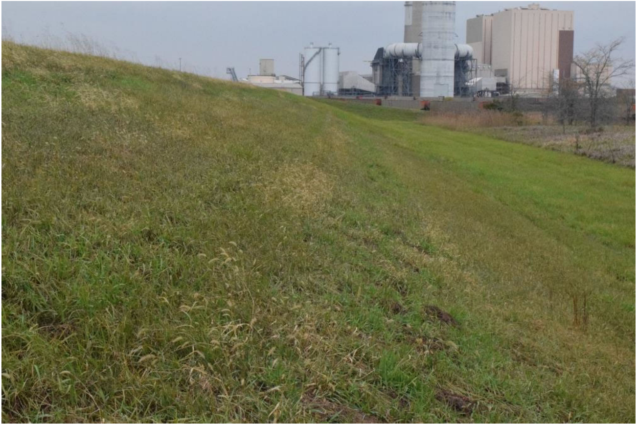
North downstream slope
