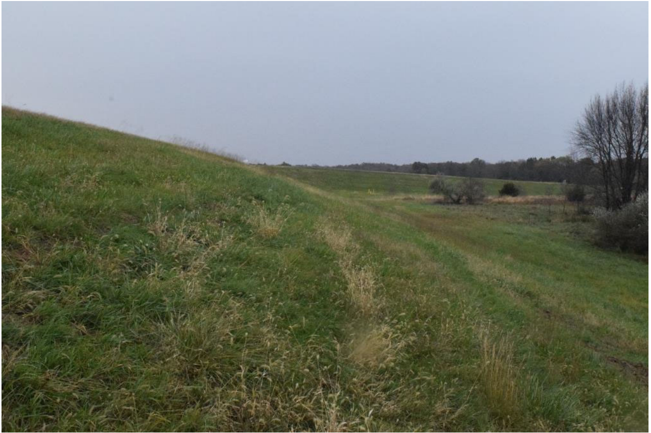
South downstream slope
