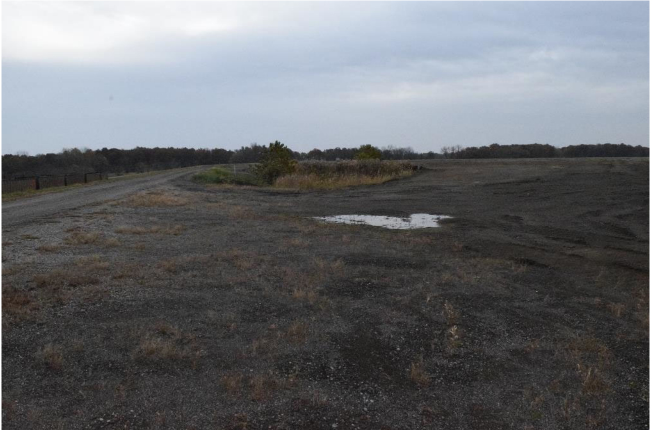
North interior and crest
