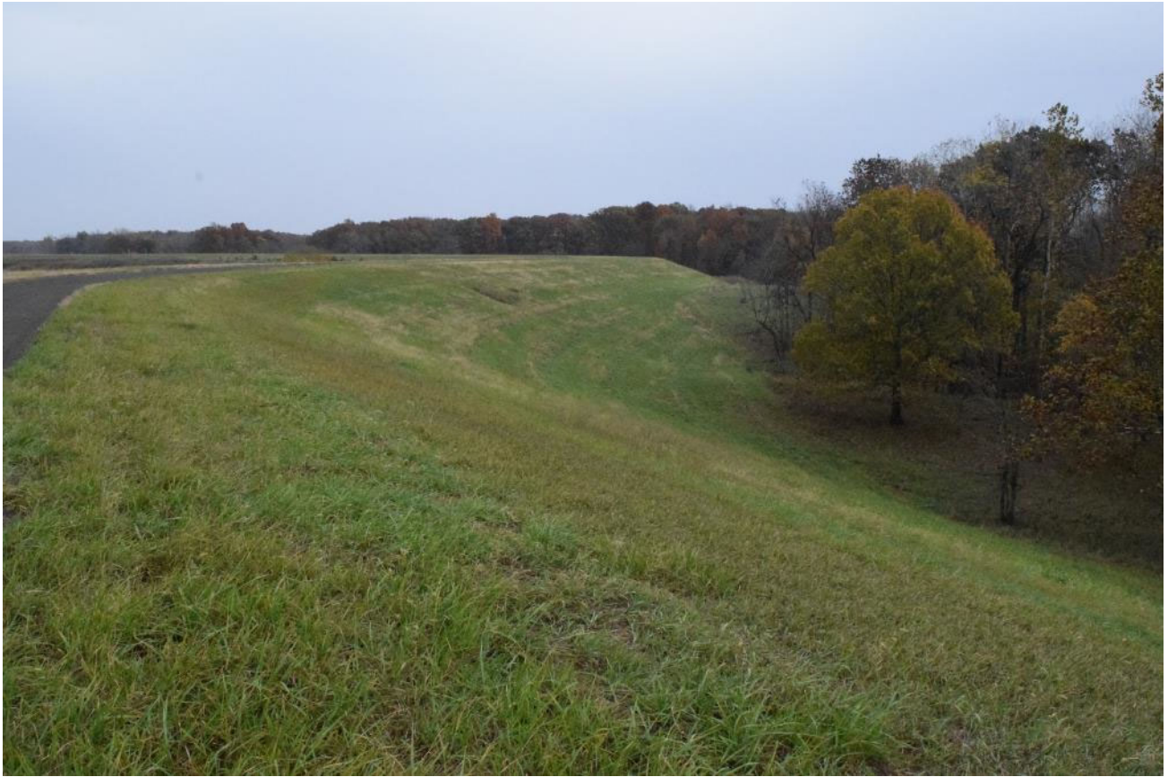
East downstream slope
